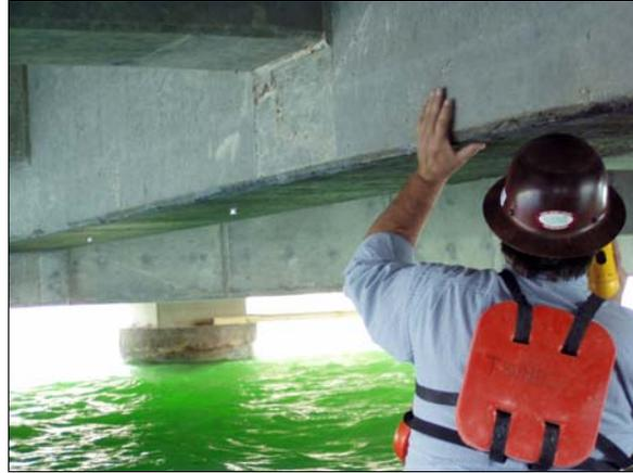
**Figure 3:** Photograph of inspector examining the FRP-concrete system
