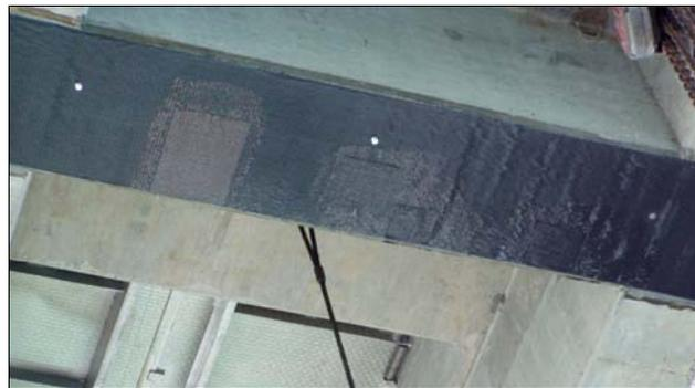
**Figure 1:** Externally bonded fiber reinforced polymer (FRP) to a concrete beam
